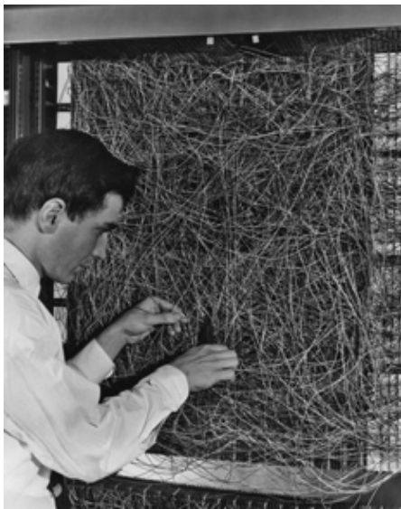
Figure 2: The Mark 1 perceptron
